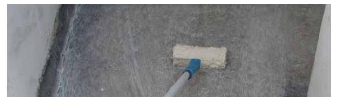
HYPERDESMO-2K-W can be applied in one single coat of 1.4kg/m2 over horizontal surfaces. On vertical surfaces this total consumption of 1.4kg/m2 can be achieved by applying 2 successive coats of 0.7kg/m2 each.
