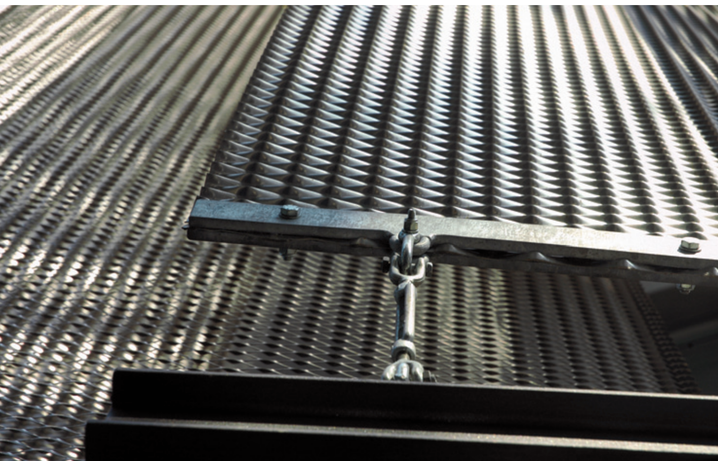
Anchoring of the strip at the bottom.
