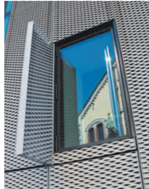
Vertical enclosure of the building, horizontal false ceiling, lateral "fins" as sunscreen for the windows to achieve the dual objective of facing and providing shade.
