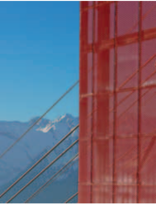
The station enclosure and its utility rooms faced in red lacquered expanded metal ensure ventilation in the rooms while providing protection against the weather and adequate illumination for the boarding platforms at the same time.
