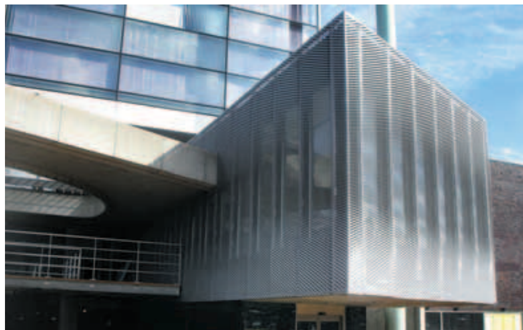
Façade in expanded metal with variable aperture mesh. Efficient sunscreen and graduated transparency that permits the adjustment of sunlight striking the glass walls.
