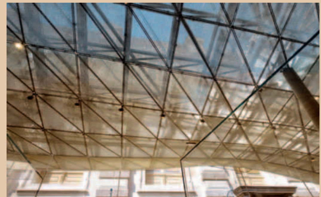
Combination of metal + glass + metal for the creation of a sunscreen with calibrated protection that filters the daylight passing through.
