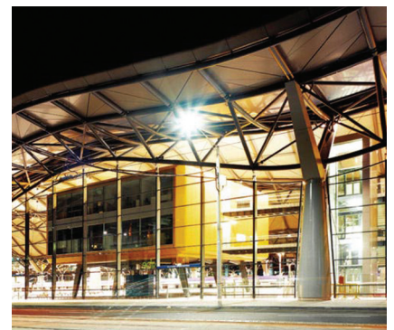
Roofing, Southern Cross Station, Melbourne, Australia
