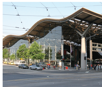
Roofing, Southern Cross Station, Melbourne, Australia
