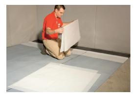
Fold an extra piece of protective foil\* (from a previous installation) in half lengthways (or cut off the equivalent of two board widths of the elastic mat to create a 'flap' of the protective foil).
