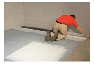
Carefully place the extra piece of folded protective foil on the exposed adhesive layer with the fold along the edge farthest from you (near the wall).\*
