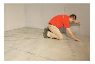
Lay the plastic moisture barrier over the screed. Make sure this is well overlapped.
