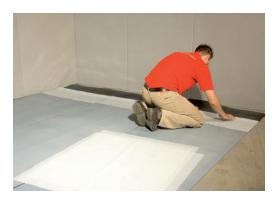
Peel back a length of protective foil equivalent to the width of two strips of flooring .
