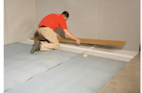
Install the first row of wooden flooring along the full length of the room. Ensuring the correct expansion joints
