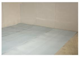
Lay the Elastic mat on top of the sheeting with the adhesive layer and protective foil facing upwards. Obviously these must not overlap.
