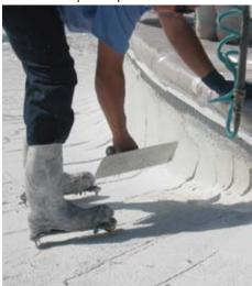
Figure 5.10 – Typical Marcite plaster installation (notice the spiked shoes).
