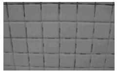
Figure 12.15 – Erosion of grout joints is the diagnosis on this application. Possible causes are as follows:
