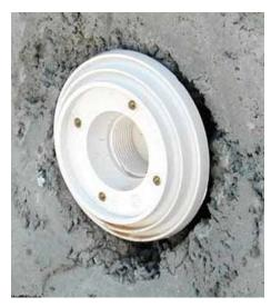
Figure 4.6 – Return port in a concrete shell pool7.
