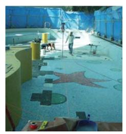
Case Study 12 – The installation of the tile in the horizontal areas is now complete. Once the tiles are installed and grouted; the installation must cure for a full 14 days after the final grouting period at 70°F (21°C) if a latex fortified portland cement based grout (e.g. LATICRETE PermaColor™ Grout) is used or 10 days if an epoxy based grout (e.g. LATICRETE SpectraLOCK® PRO Grout\*) is used.
