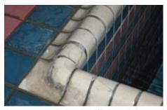
Figure 7.6 – Uniquely shaped pool/deck rim which required careful forming of the render in order to place the finished tile.
