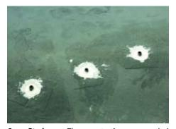
Case Study 9 – The penetrations are sealed with a suitable flexible sealant. Generally, 100% silicone sealant (e.g. LATICRETE® Latasil™ with LATICRETE 9118 Primer) or urethane sealant with non-solvent based primers can be used. All precautions to create a complete watertight tank must be taken to ensure a successful flood test.
