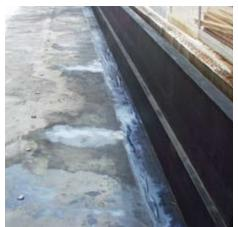
Figure 12.2 – Effects of exposure to rain prior to the waterproofing membrane reaching its full cure. This damaged waterproofing membrane will need to be removed, reinstalled, protected and allowed to reach its full cure.
