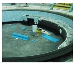
Case Study 11 – The tile installation can now begin. Generally, work begins on the vertical areas first. A high strength liquid latex fortified thin set mortar (e.g. LATICRETE 254 Platinum; or, LATICRETE 4237 Latex Additive mixed with LATICRETE 211 Powder) suitable for submerged applications is used. Care is required when working over the waterproofing membrane.
