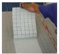
Figure 12.7 – Porcelain mosaic tiles installed on pool deck. Notice the ribbons of latex fortified thin set mortar combed in one direction to maximize coverage.
