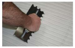
Figure 7.1 – Trowel applied medium bed mortar with a 3/4" (19 mm) loop notch trowel.
