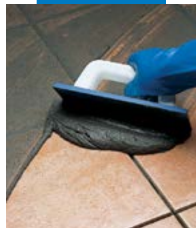
Grouting single-fired tiles with a float
