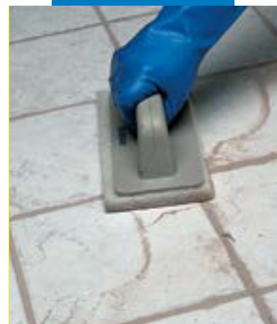
Finishing with a Scotch-Brite® pad
