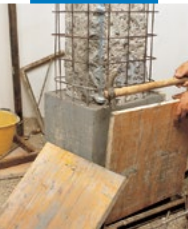
Removing wooden formwork
