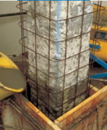
Pouring into a formwork
