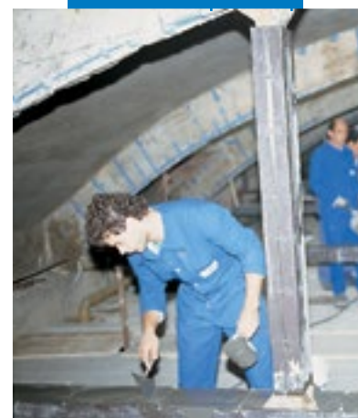
Pouring Mapegrout Hi-Flow ZA into metal formwork
