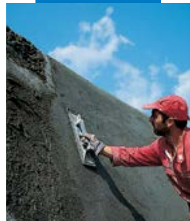
Finishing of Mapegrout T40
