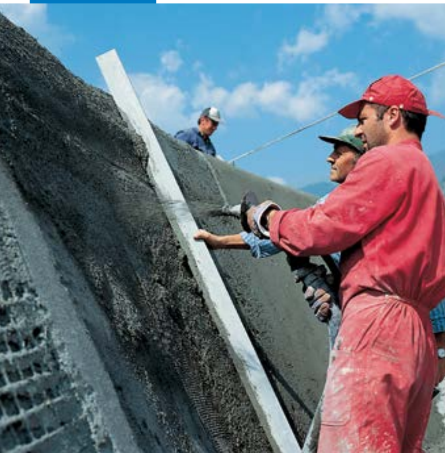
Spray application of Mapegrout T40
