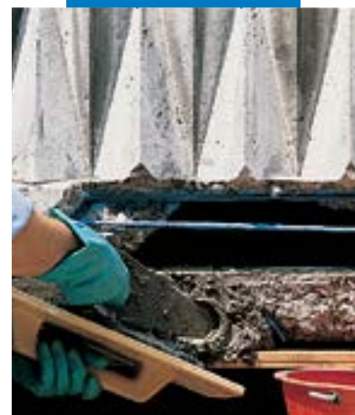
Repairing a balcony with Mapegrout T40
