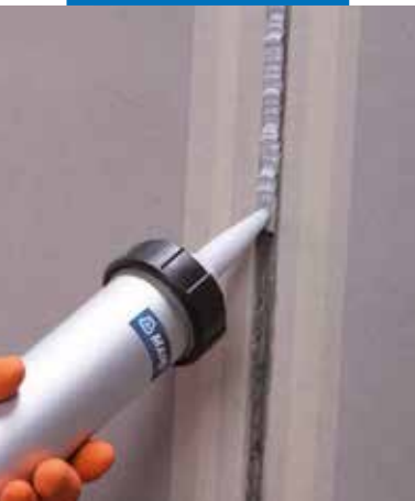
Application of Mapeflex PU40
