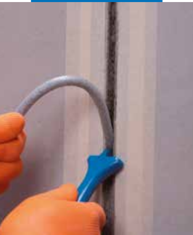
Inserting Mapefoam inside the joint
