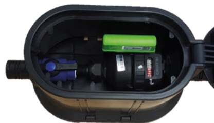
GROUND LEVEL BOX WITH SABS BALL VALVE AND WATER MANAGEMENT DEVICE (WMU)
