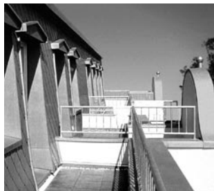
Fig. 30: RHEINZINK-flashing as a wall coping
