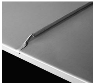
Fig. 16: Ridge as eave termination
