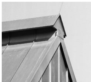
Fig. 17: Flush ridge termination on verge, high design
