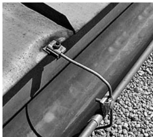
Fig. 14: Incorrect installation of lightning rod terminal to panel
