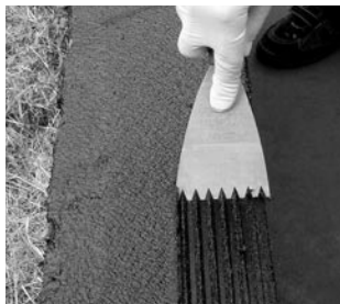
Fig. 5: Apply Enkolit® with notched trowel
