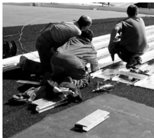
Fig. 10: Structured mat without underlay, Enka®-Vent
