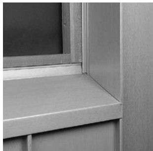
Fig. 26: Jamb on lateral connection windowsill coping
