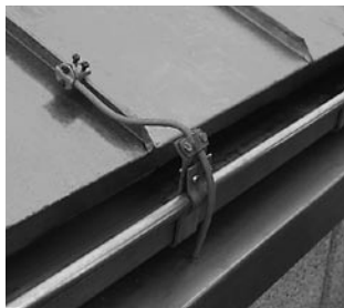
Fig. 13: Proper installation allows for thermal expansion of panel
