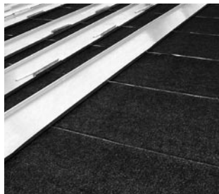
Fig. 9: Structured underlay, installation above wooden sheathing
