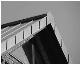
Fig. 18: Flush seamed ridge termination on verge fascia, low design
