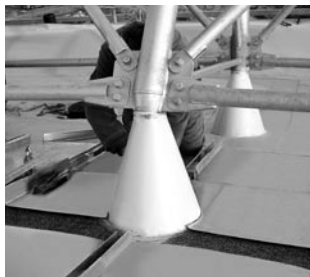
Fig. 7: Roof area with many penetrations
