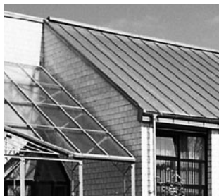
Fig. 15: Pent roof ridge
