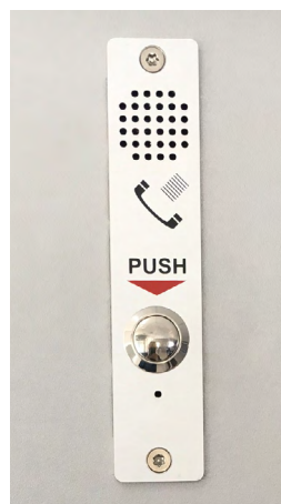
EXTERNAL SIDE PUSHBUTTON, TRAFFIC LIGHTS & INTERCOM
