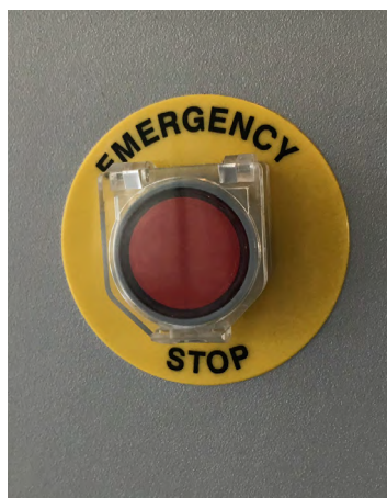
INTERNAL EMERGENCY PUSHBUTTON
