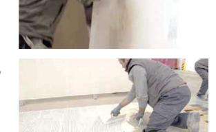
Using the appropriate sucker frame, position the slab on the adhesive bed, being careful to maintain a minimum joint of 3 mm.
