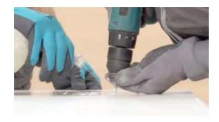
To drill internal cutouts from the slab, you need first of all to draw the guide lines.
