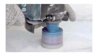
Round holes must be made in wet drilling, using diamond blades.
