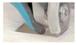
Follow the drawn lines using a diamond blade angle grinder and then finish off the edges with a diamond polishing pad.
