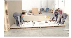
Complete the laying operations using a suitable sealant, while keeping at least a 3 mm joint through the use of spacers. To make the task easier, use the special device for pulling over the slabs, available on the market.
