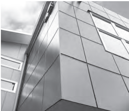
LEFT External fitout in modular form: Weathergroove 1200 Pre-Primed and painted, off-stud installation. Cut panel heights of Weathergroove to custom sizes to create a panelised or bricklaid patterns.
