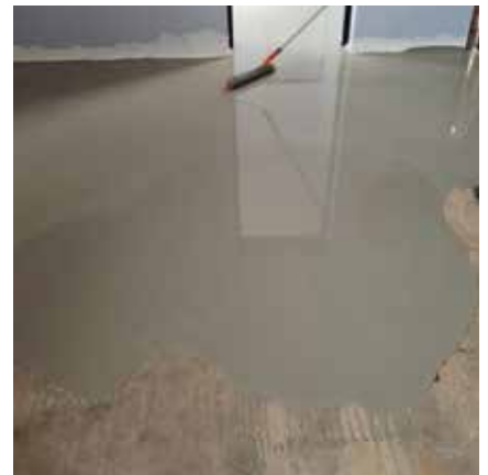
abe.®screed SLC acrylic primer used with abe.®screed SLC P Project - receive vinyl flooring
