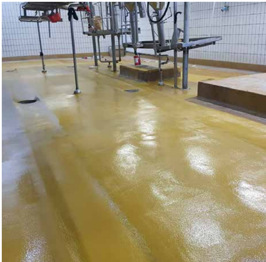
Beefmaster Abattoir Kimberley abe.®prime GCP (Green Concrete Primer) used with abe.® screed PU
