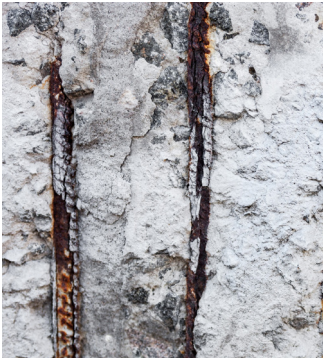
Corrosion is an irreversible chemical reaction that, if left unattended, actually accelerates over time and develop cracks, concrete delamination and, eventually, spall their concrete cover to expose severely degraded steel.
