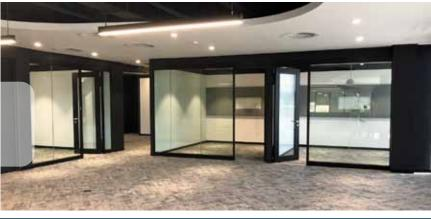
The GF Serene Range integrates directly with the Aluglass Bautech Varikust® VK62 acoustic doors.
