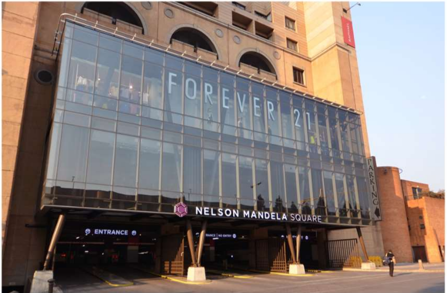
Flush Glazed Curtain Walls @ Nelson Mandela Square
