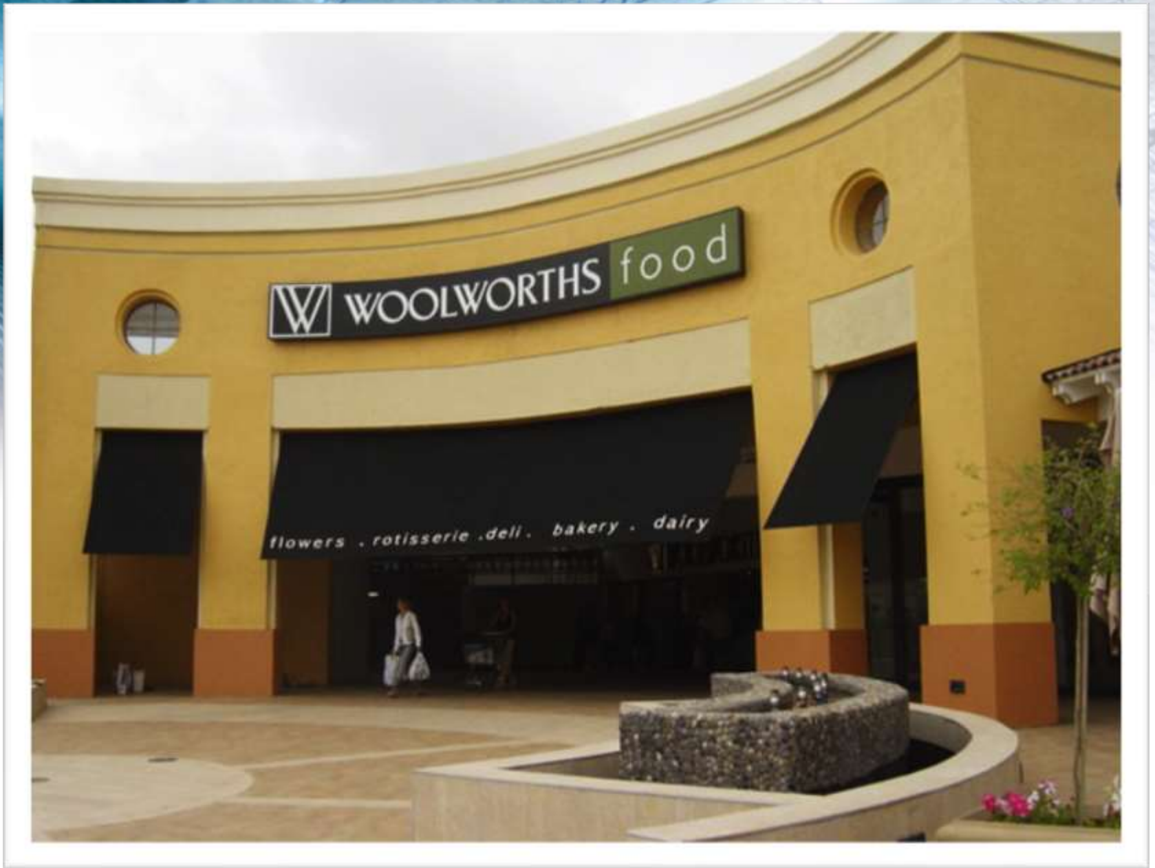
Solamark® fixed screen awnings @ Lonehill Shopping Centre
