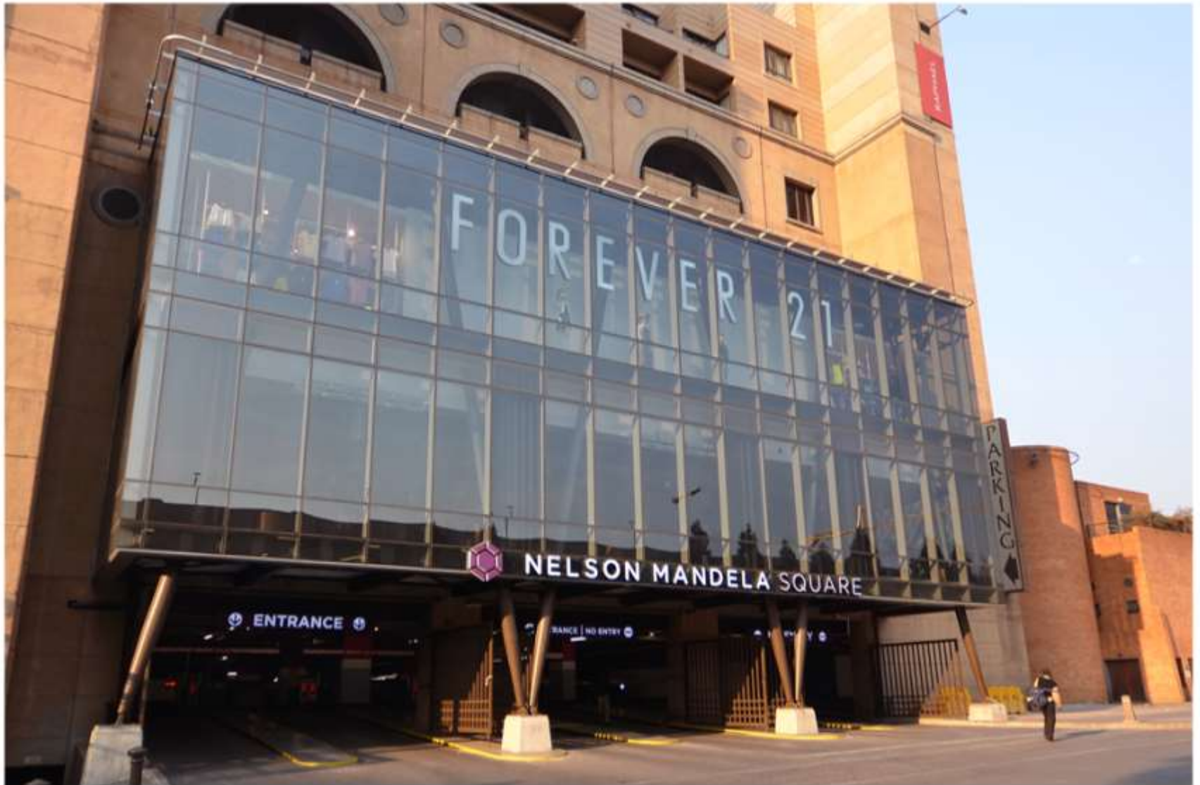
Flush Glazed Curtain Walls @ Nelson Mandela Square
