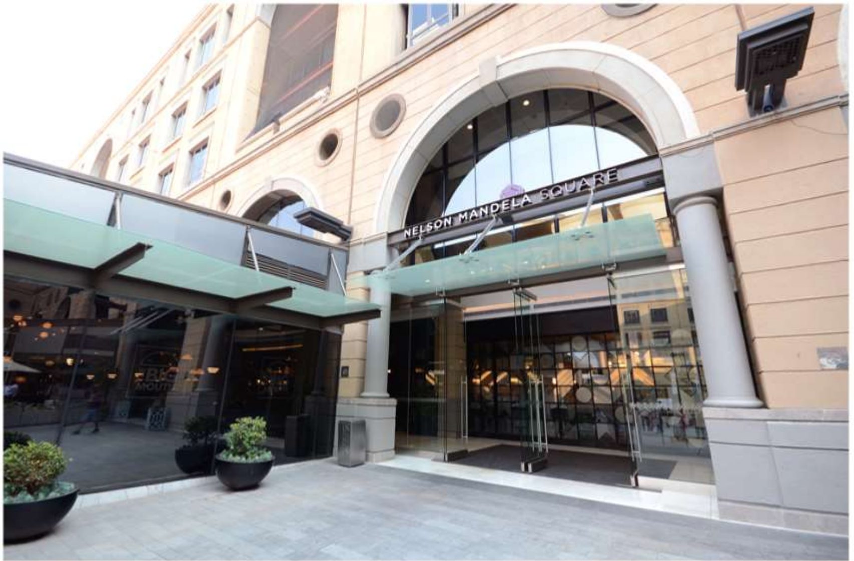
Frameless Glass Entrance Doors and Canopy Glass @ Nelson Mandela Square
