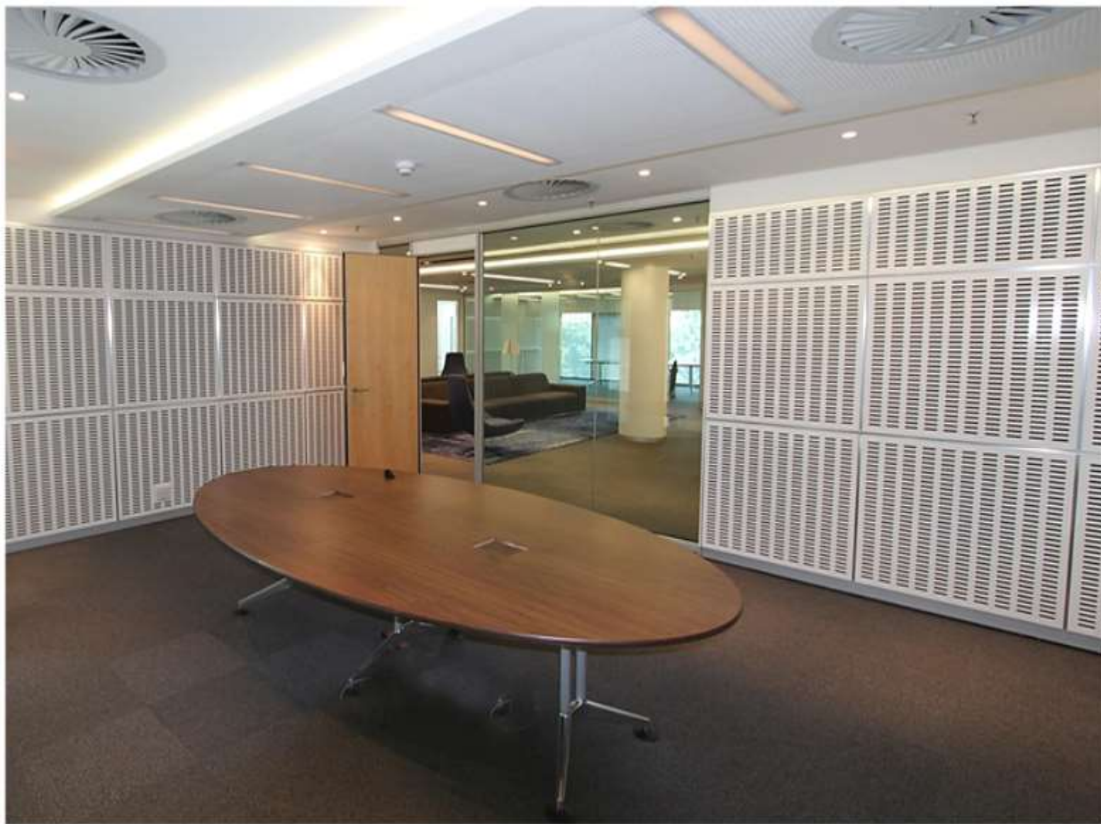
Absorption Panels, GF Serene and Varikust doors @ Deutsche Bank
