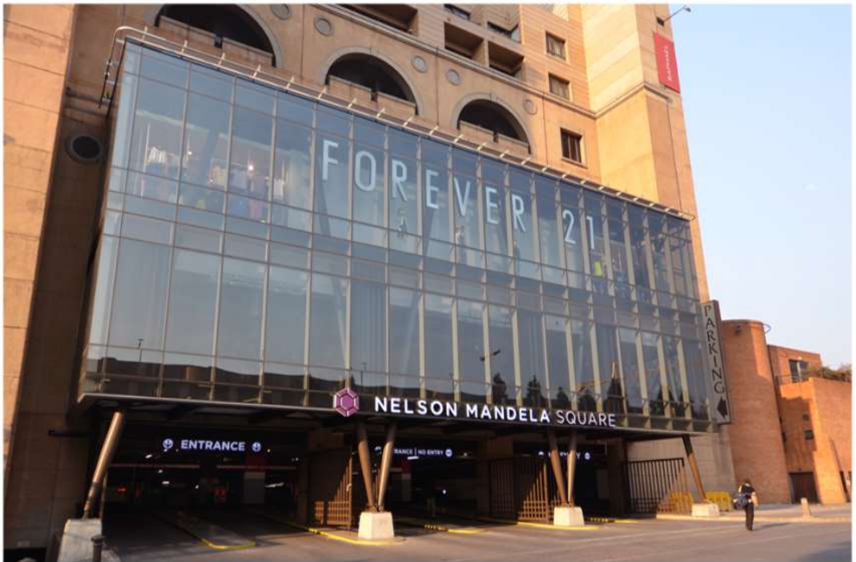
Flush Glazed Curtain Walls @ Nelson Mandela Square
