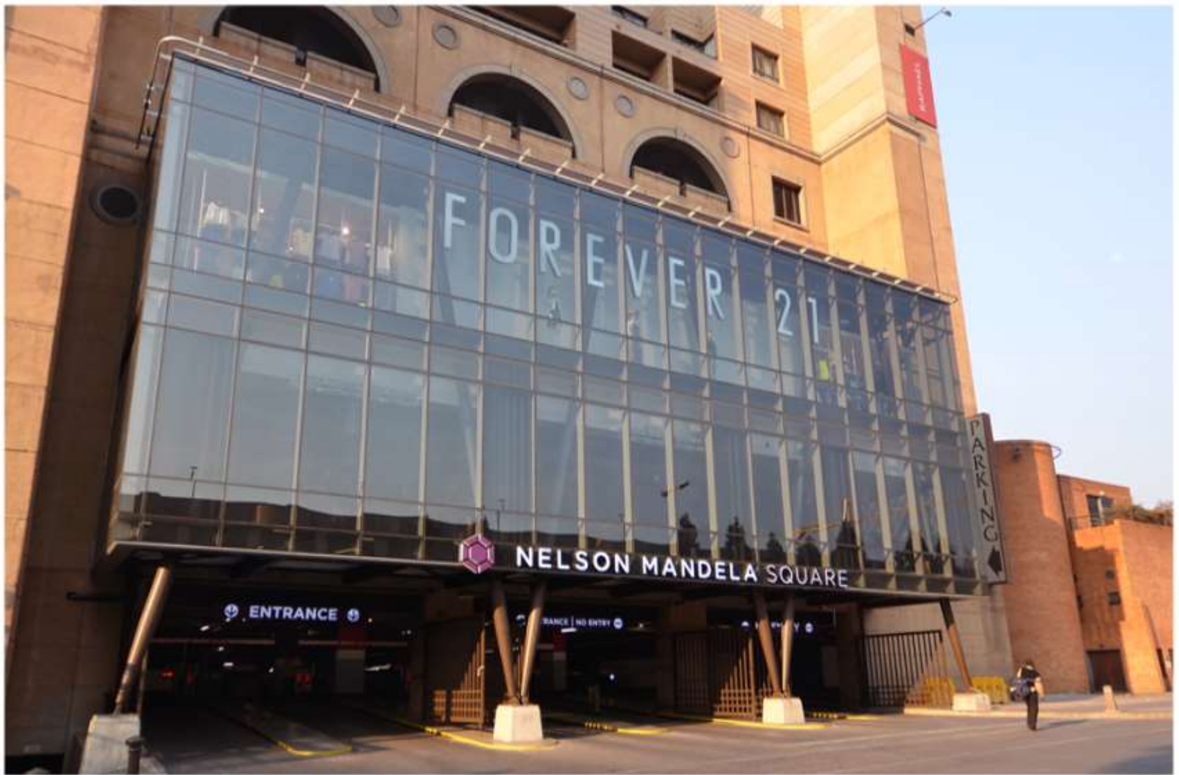
Flush Glazed Curtain Walls @ Nelson Mandela Square
