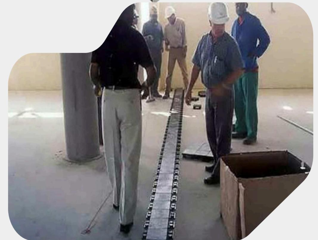
Using a chalk line make sure the first line is straight, then having completed this start a new line from the central point at 90 degrees to the first line and ensure that this line is straight
