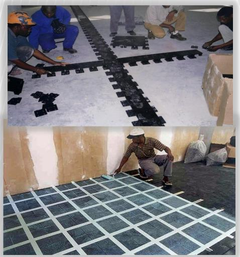
Cyberfloor installs as easily as laying carpet. The system allows for maximum flexibility and adapts easily to all spaces. Any flooring finish can be selected for use with Cyberfloor, however, we suggest a good contract carpet that complies with fire grade SABS 0400.
