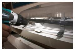
Secure dome carefully against 2<sup>nd</sup> brackets with tech screws & rubber washers (hole in perspex dome to be pre-drilled slightly larger than shaft of fastener)
