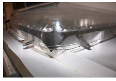
Corner view (note rubber seal is pushed downwards at outer edge when dome is placed in position).
