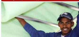
Saftherm™ polyester blanket insulation cut and snugly placed in the ceiling void between the trusses.
